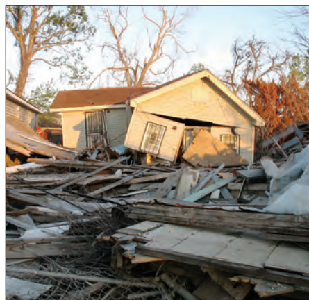
An example of the destruction of Hurricane Katrina.
