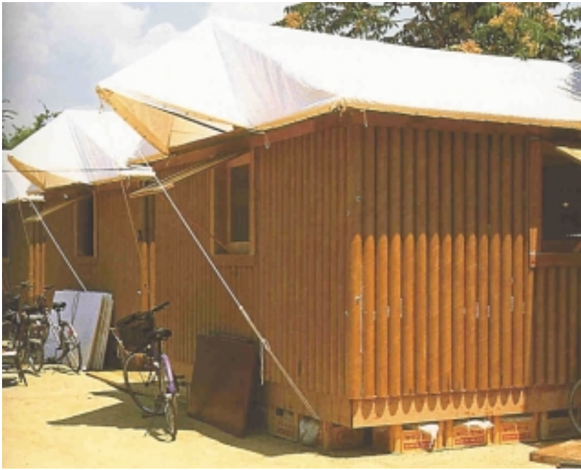
Paper Log House, Kobe, Japan, Shigeru Ban Architects, © Takanobu Sakuma.
