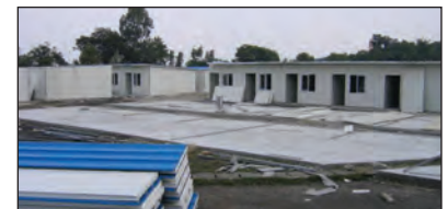
During summer 2008, 324 temporary housing units for faculty and staff were built on athletic fields, wrote SWUST English professor Xiong Tingting by email. The 215-square-foot units fit two to three people. Communal bathrooms, one for every 10 units, don't have water heaters. Some 200 units are occupied. Older staff quarters – about 3,000 units – were demolished. New permanent buildings are under construction. It will take at least two years for them to be ready. (July 2008 photo by Steven Plummer.) ■
