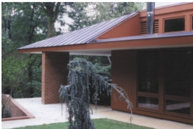
New wing and courtyard, Kamphoefner-Petrocella House. Robert Burns, photographer, 2002.
