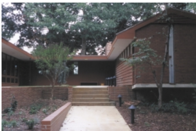
New entryway, Kamphoefner-Petrocella House. Robert Burns, photographer, 2002.
